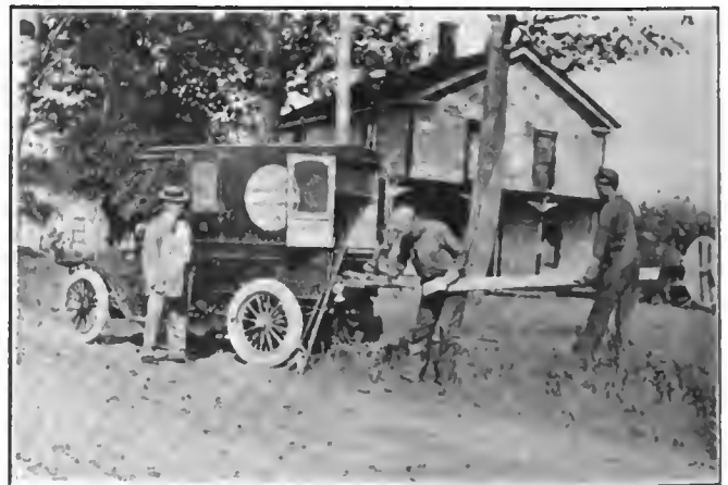
Nailing on the Timber Cross Piece
